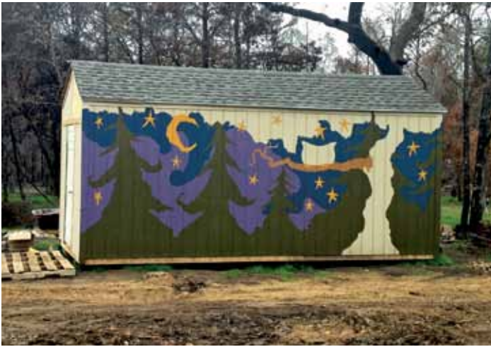
Before Extreme Makeover: Home Edition knocked on their door, this shed was going to serve as the Zdroj family home.
